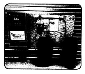
Anolyte generators produce the disinfectant through an electrolysis process using salt and water. This technology ensures employees always have the necessary cleaning solutions on hand and that all facilities are properly and frequently cleaned, without exposing individuals to toxic chemicals. Once installed, a generator produces a 500 ppm HOCL solution for as low as \$0.04 per gallon.
